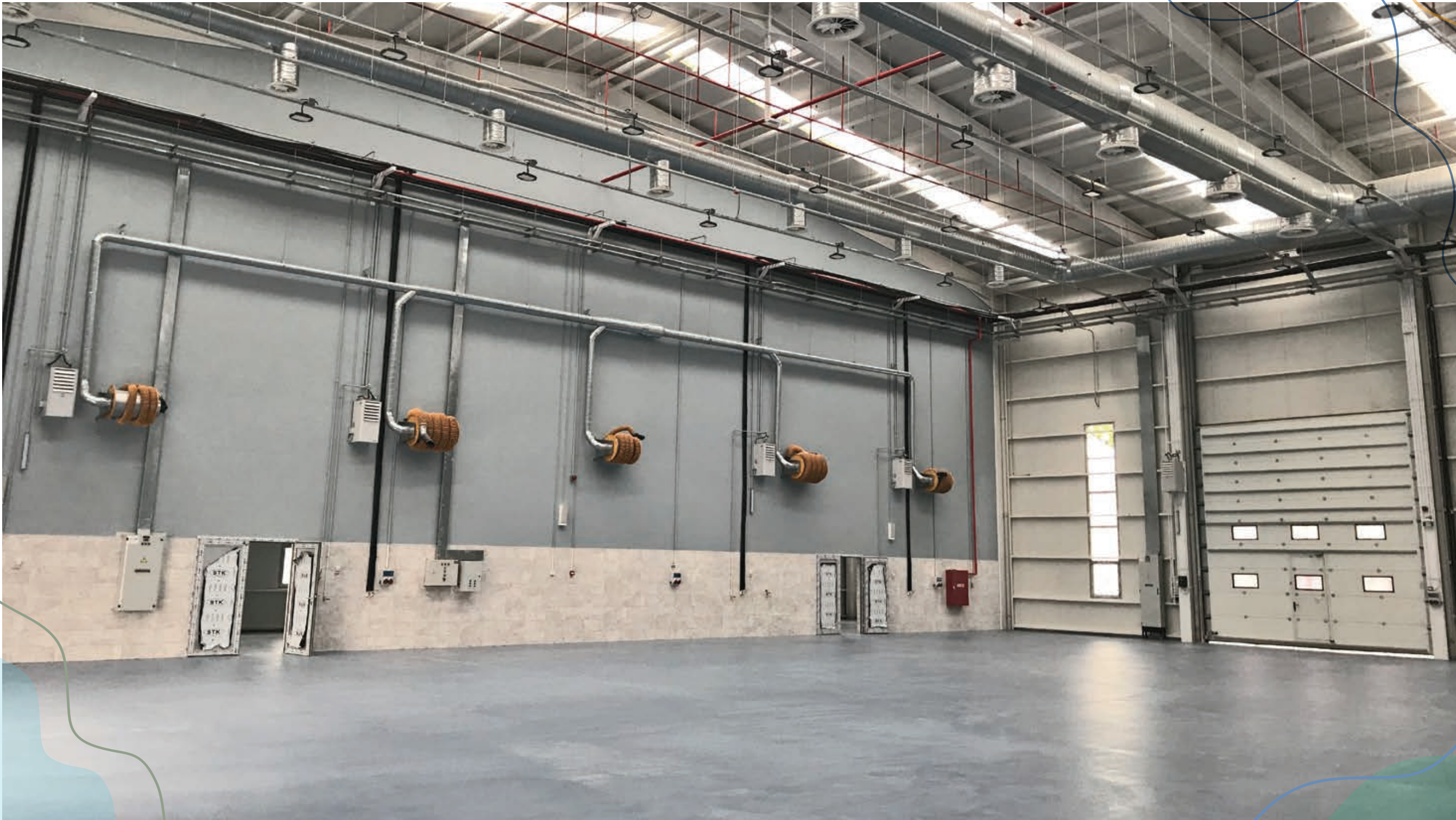
ESENBAGA AIRPORT MAINTENANCE BUILDING
