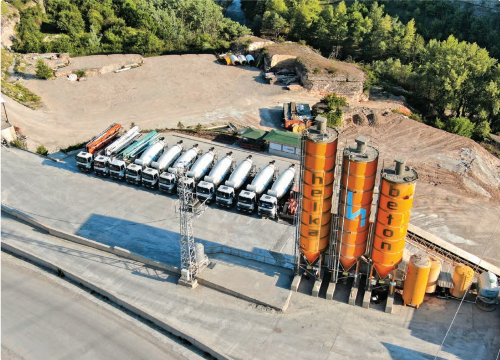
KARABÜK CONCRETE PLANT
