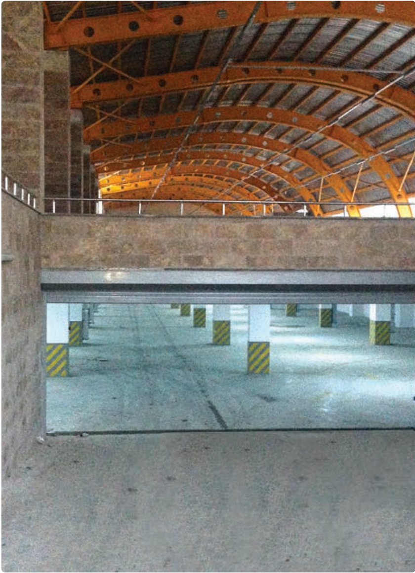
ERBAA PARKING LOT / 2013
